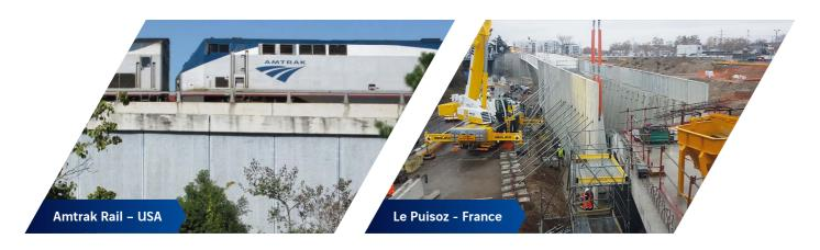
TechWall™ relies on counterforts, which play a crucial role in ensuring the overall stability and strength of the retaining wall. By acting as cantilever beams, the counterforts can effectively resist the lateral earth pressure, thereby reducing the moments in the facing panel. As a result, the thickness of the concrete panel can be minimized, without compromising the strength and durability of the structure.
