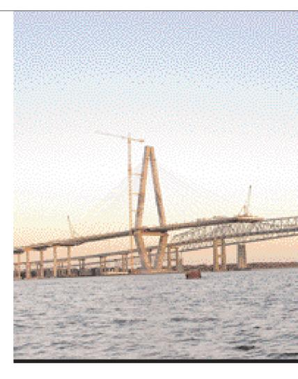
struction works, we had to erect "high-wind" stability cables to stabilise the structure when the average wind speed exceeded 75 km/h for an hour. Thanks to a system made up nails and a counterweight, the deck swung like a pendulum during the hurricanes.
