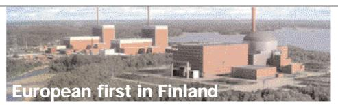
A member of the consortium responsible for building the first EPR (European Pressure Reactor) nuclear reactor on the Olkiluoto site in Finland together with Siemens, the Areva Group has entrusted the supply and implementation of the prestressing of the protective shield to Freyssinet's Structures division. After the Tianwan nuclear power plant (China), this will be the third protective shield that uses Freyssinet 55C15 prestressing anchors.
