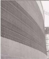
made up of 4 strands each 138 m long connected by 468 X anchors, enclosed in single HDPE ducts injected with cement grout.
