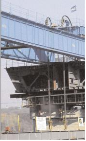
In association with supply and installation of the stay cables and heavy lifting, Freyssinet was also involved in a third part of the project: installation of bearings and use of out-of-specifications systems. In this respect, the structure also broke a third record. Of the 56 bearings installed on the piers, two spherical bearings, one placed on each of the end piers, were of extraordinary dimensions and had a nominal capacity of 110 mN.
