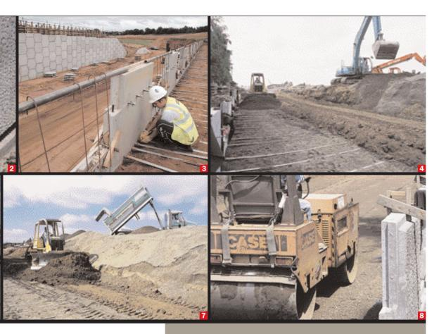
Prefabricated facing scales (1,3), metal or synthetic reinforcements (4,7), backfill material (4,6,7,8): the components of the technology place Reinforced Earth halfway between geotechnics and structures. After they have been laid, they form a composite material that is durable, effective and able to adapt to the most complex configurations.
